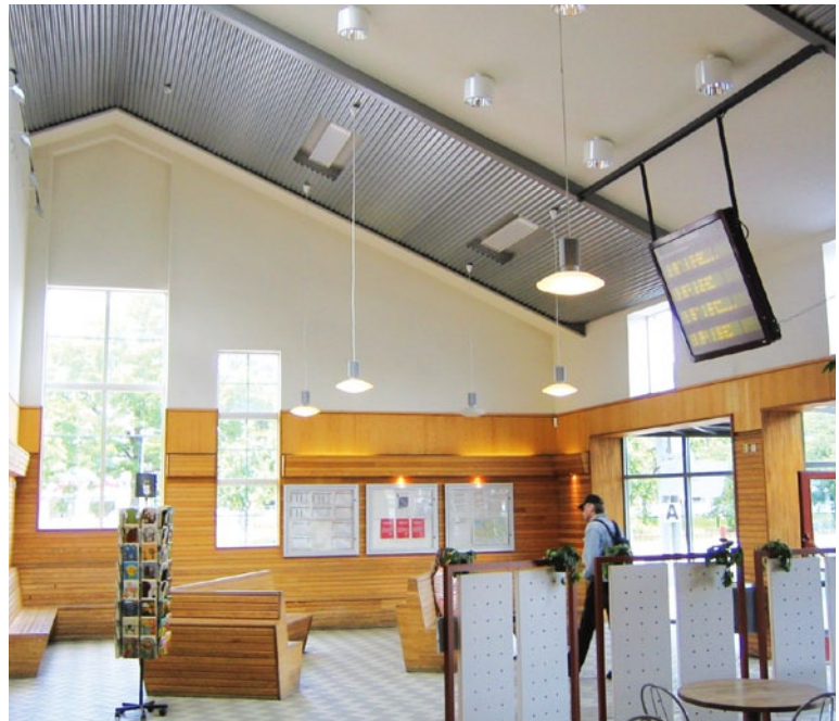
The nice wooden walls are kept free with EZ100 mounted on the ceiling.
