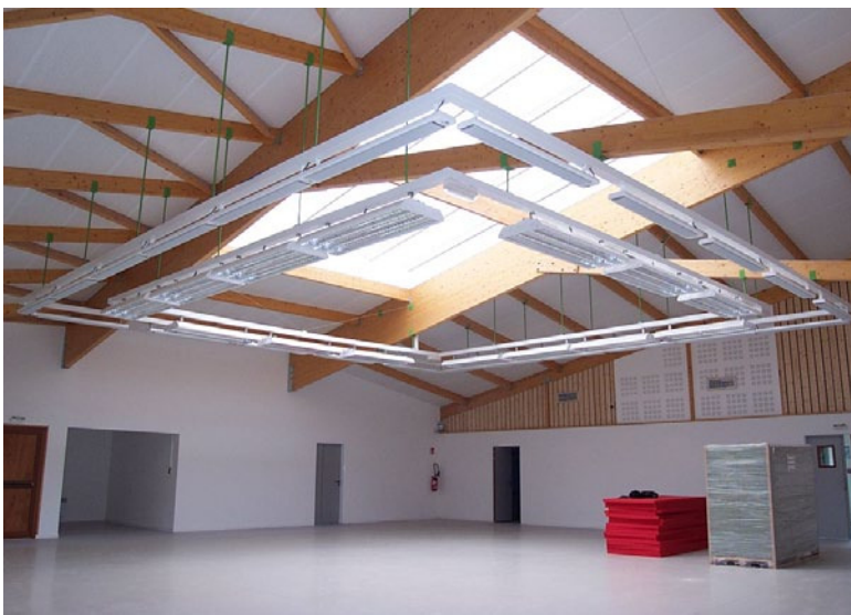
Buildings that are used on an irregular basis can be heated fast without a high energy consumption. EZ100 blends well with electrical fittings.
